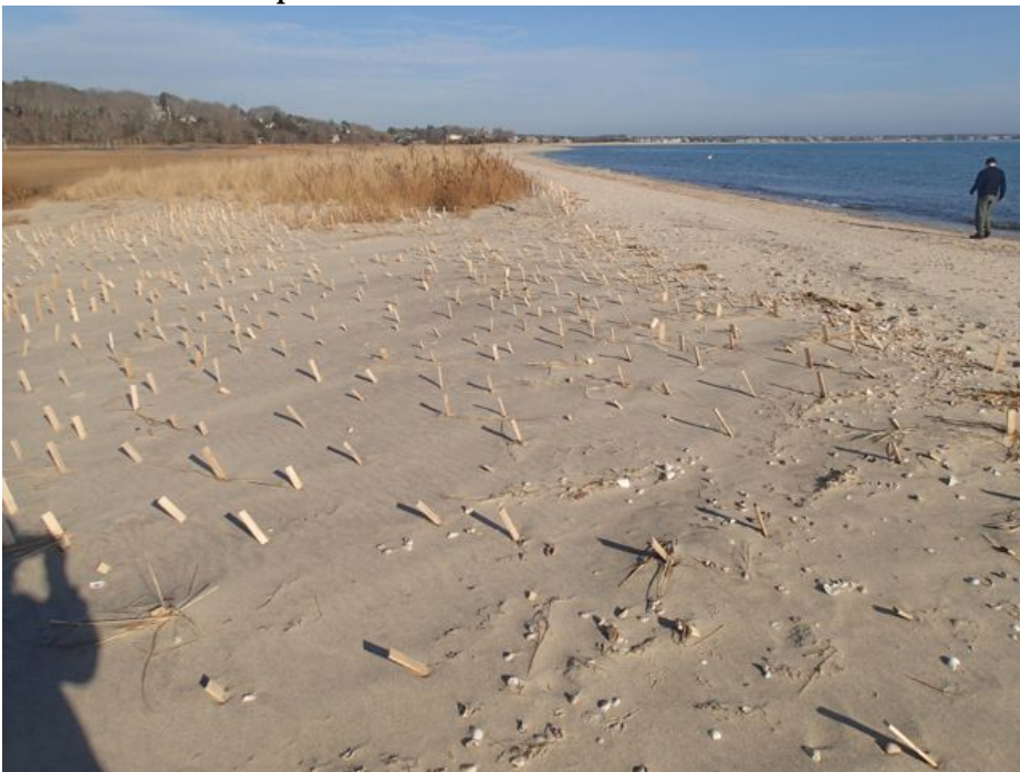
Nearly 2 feet of new elevation was established during the storm season, providing a lower risk platform for replanting of American Beach grass.
