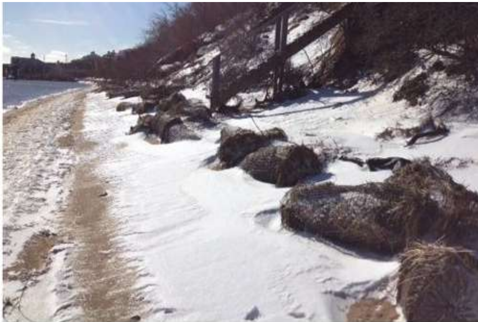
Image by Kayla Anderson, Safe Harbor. Detached coir following storm event may impact adjacent or downwind beaches and may remove vegetation while being washed ashore.
