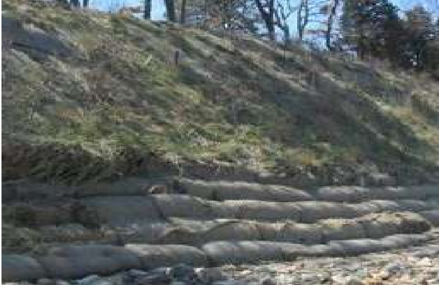
Image by G. Peabody. Storm events remove nourishment, exposing coir.
