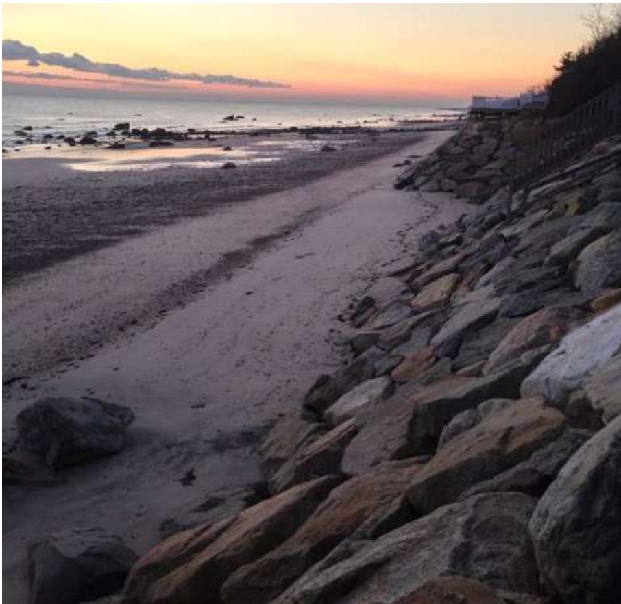
Image by G. Peabody. Revetments impact the coastal process by interrupting bank-to-beach sediment flow. The stones should be covered with nourishment and renourished when storm energy removes the sand. This has impacts on alongshore sand transport.
