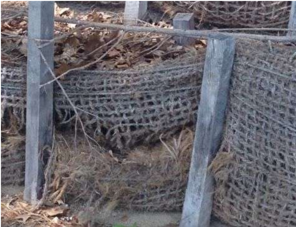
Image by G. Peabody. Exposed step blocks are vulnerable to deterioration.
