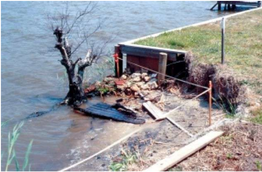
Image above: Classic “End Scour” from redirected wave energy and failure to nourish.
