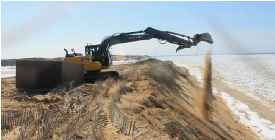
Image by G. Peabody. “Full bank” nourishment. To reduce impact, sand is delivered to dump box from sand storage area. Application equipment transfers nourishment laterally and diagonally from planned transfer areas along the full height of the bank. Full bank nourishment provides longer term, more sustainable, protection.
