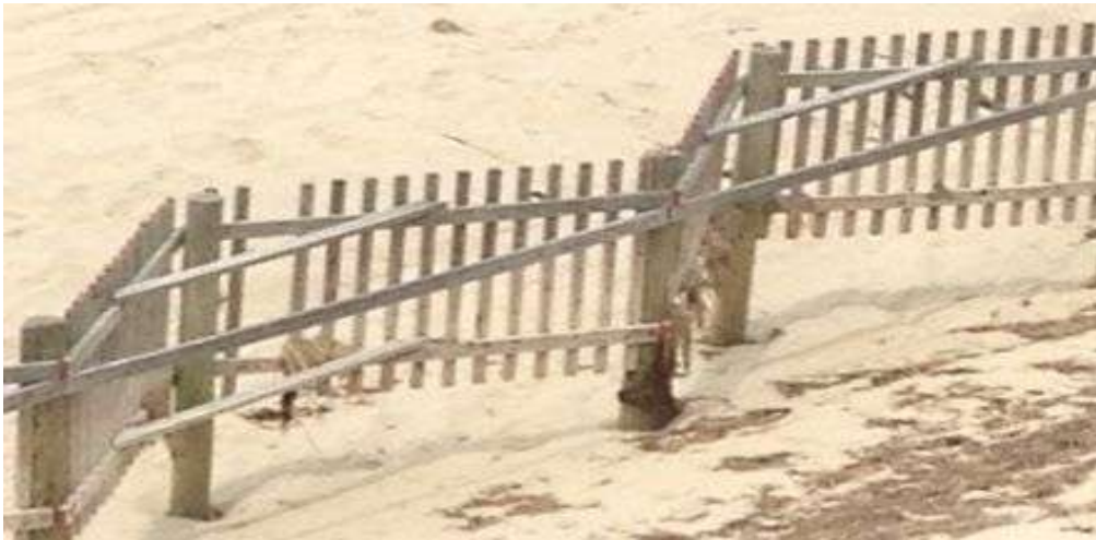
Image by G. Peabody. Sand loss seems unaffected by drift fence.
