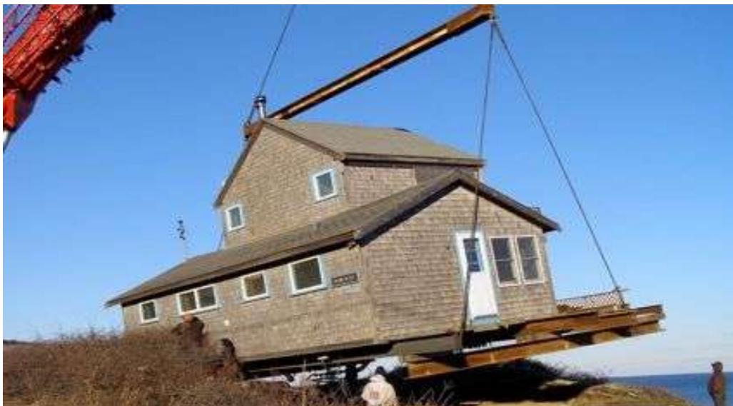
Image above by G. Peabody. Retreat: Relocating a residence away from a coastal bank.
