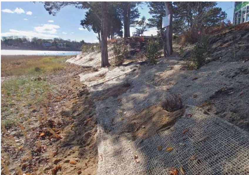
Image by G. Peabody. Affordable Jute provides temporary surface stability.
