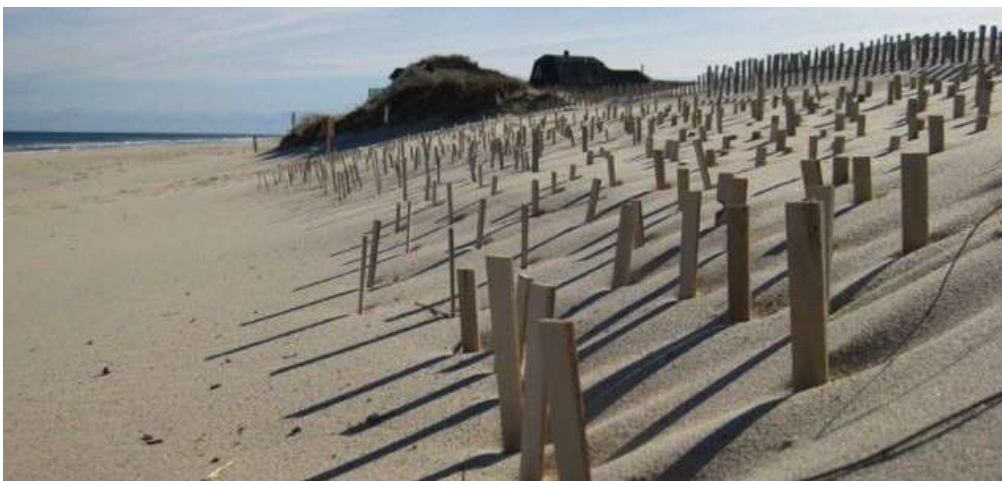
Image by G. Peabody. Safe Harbor's minimal, random matrix, restoration system. As storm blown sand collects, the shims can be lifted up higher to control sand collection platform. Collection rates vary based on nearby sand supply.
