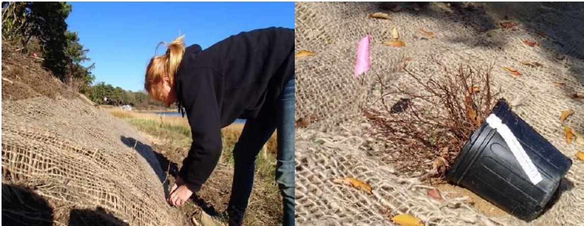
Images by G. Peabody. Jute netting easily accommodates plantings of soft stem and woody stem Native vegetation. Cornstarch staples secure jute net.
