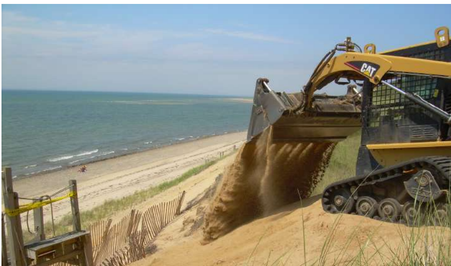
Image by G. Peabody. Nourishment can be sourced from adjacent foundation excavations.
