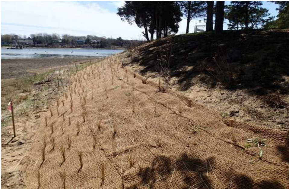
Image by G. Peabody. Heavier mats mark the change between lower and higher effort sand cladding systems because they need labor-intensive securing systems.
