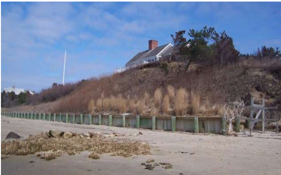
Image by G. Peabody. Bulkheads change erosion patterns on site.
