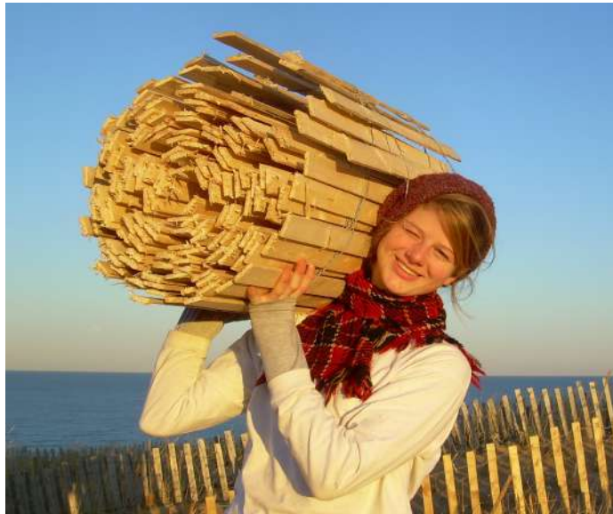
Images G. Peabody. Rubber mallet installation. 4' roll cut in half provides 100' -24" fence.
