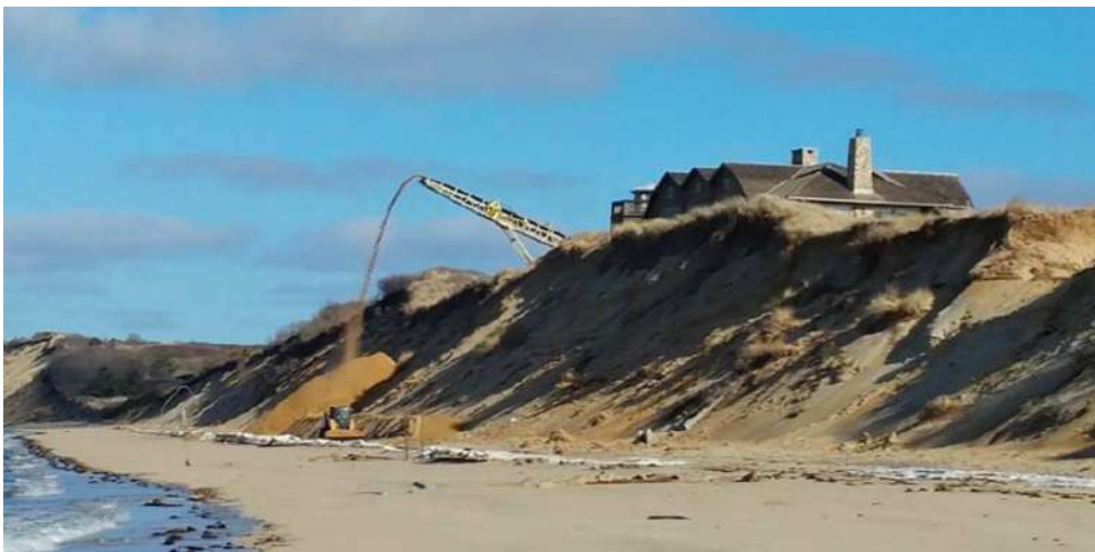
Image by Safe Harbor. Conveyor being used to deliver sand to toe of bank.
