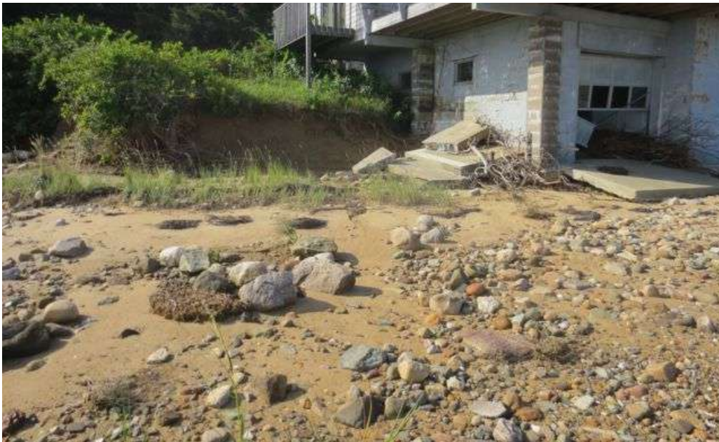
Image by G. Peabody. This home, subject to changing storm surge levels, was being destroyed by wave action.
