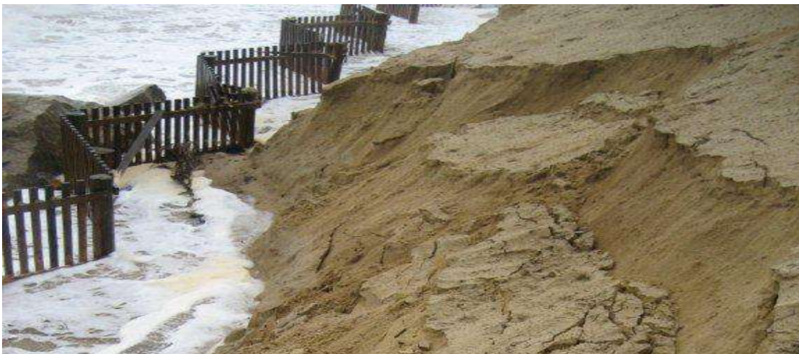
Image by G. Peabody. Drift Fence may restrict overwash outflow, contributing to outwash of sand.
