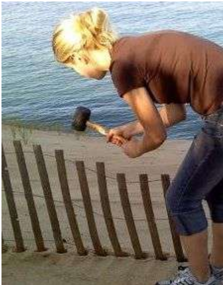
Images G. Peabody. Rubber mallet installation. 4' roll cut in half provides 100' -24" fence.
