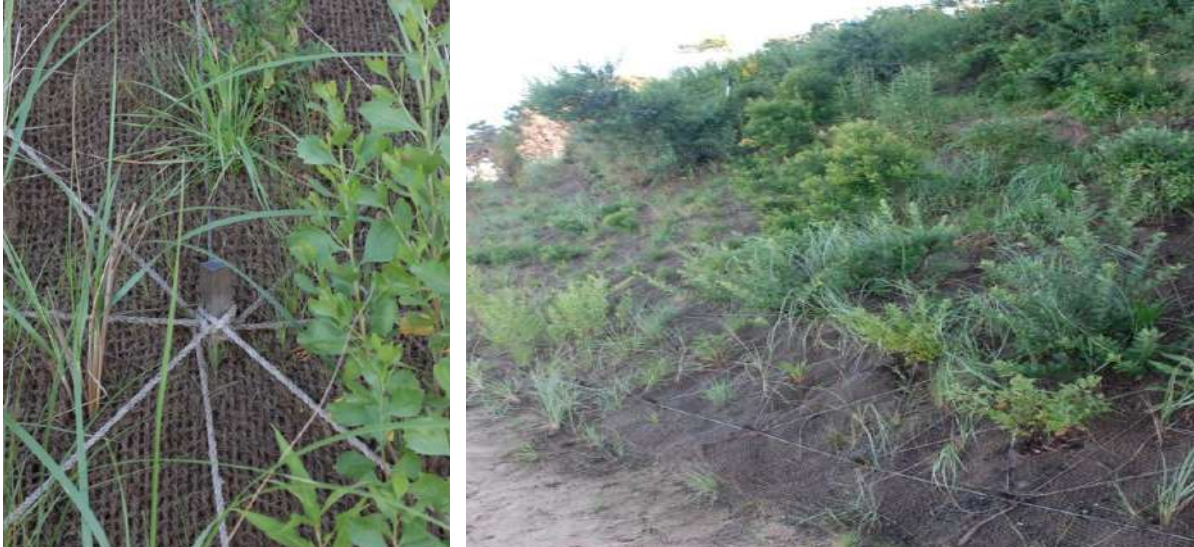
Images by Andrew Barr. Vegetation, stakes and cables secure Geo Mat over coir.
