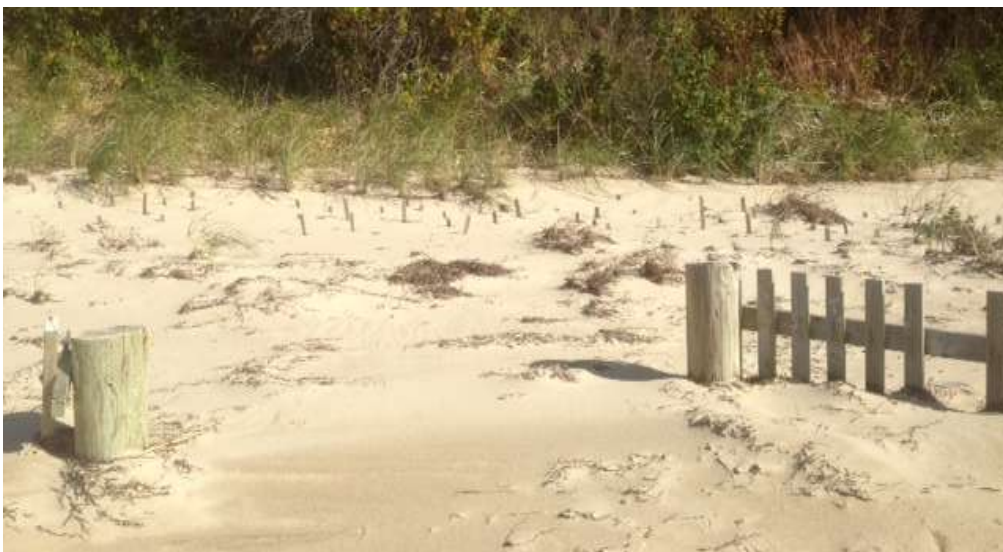
Image by G. Peabody. Sand accumulation seems unaffected by drift fence.
