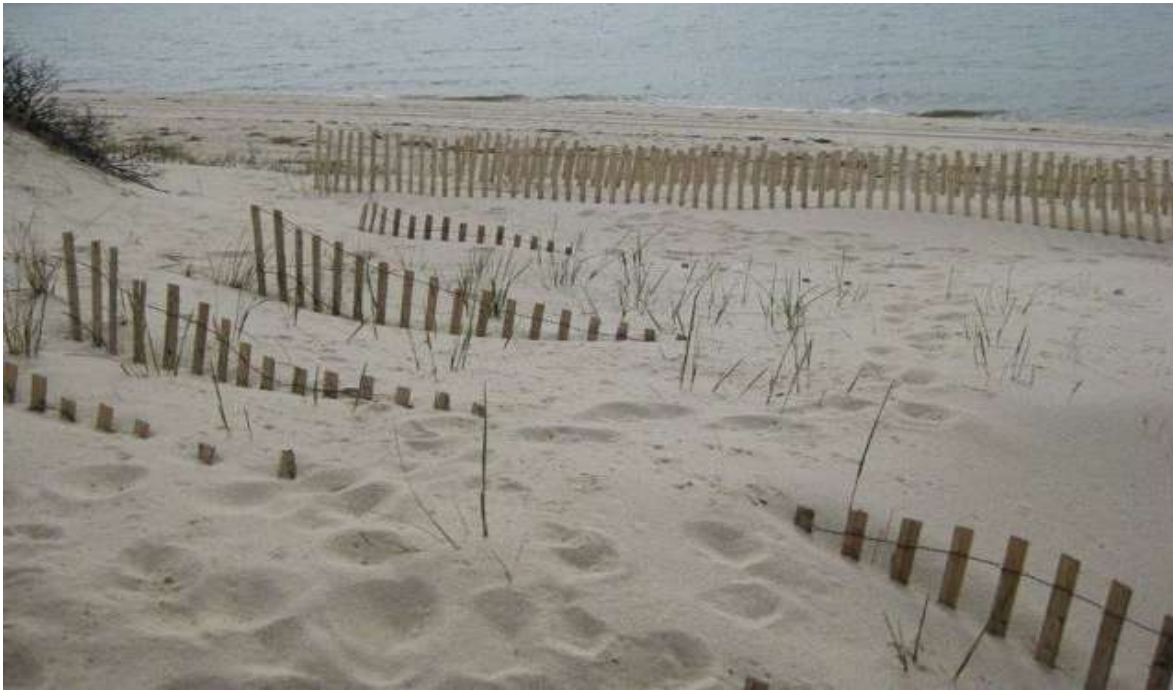
Image G. Peabody. 24" Sand fence at Bayside restoration site, works with wind energy.
