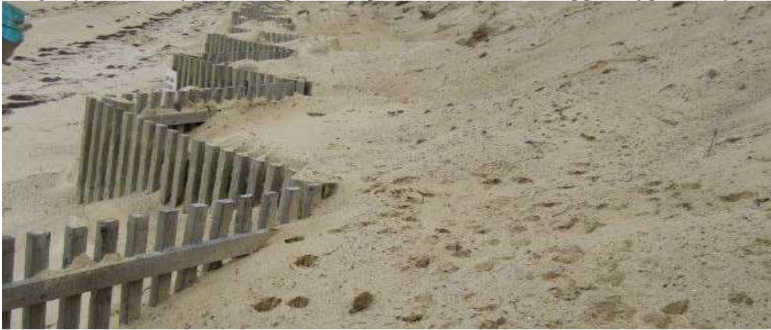
Image by G. Peabody. Drift fences also require sand nourishment and beach grass planting.
