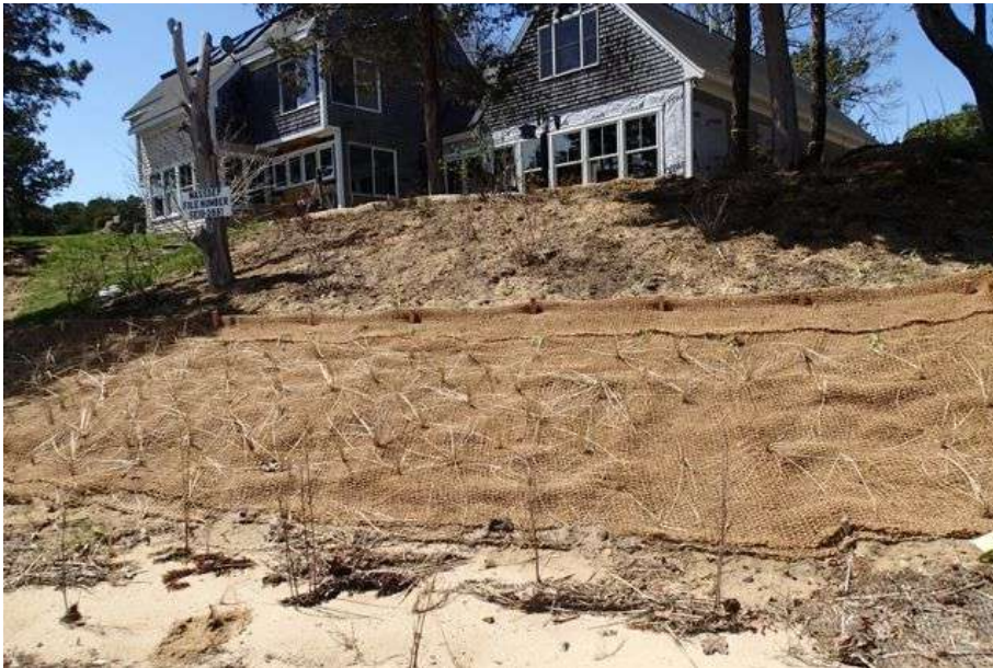
Image by G. Peabody. Geo Mats are prone to bunching if not well secured.
