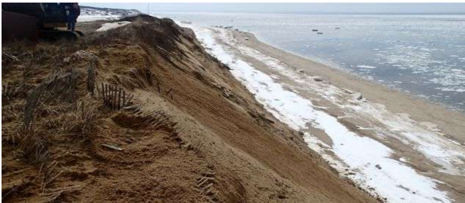
Image by G. Peabody. Full bank nourishment is most effective when possible.
