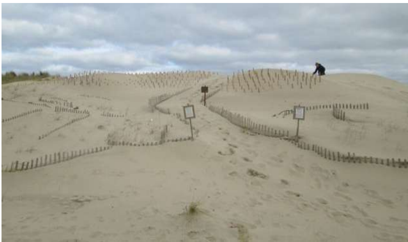
Image G. Peabody. Biomimicry barrier dune restoration before planting. Dune gained approx. 10-12 vertical ft./yr. Zig-zagged pedestrian pathway provides access and prevents wind blow outs.
