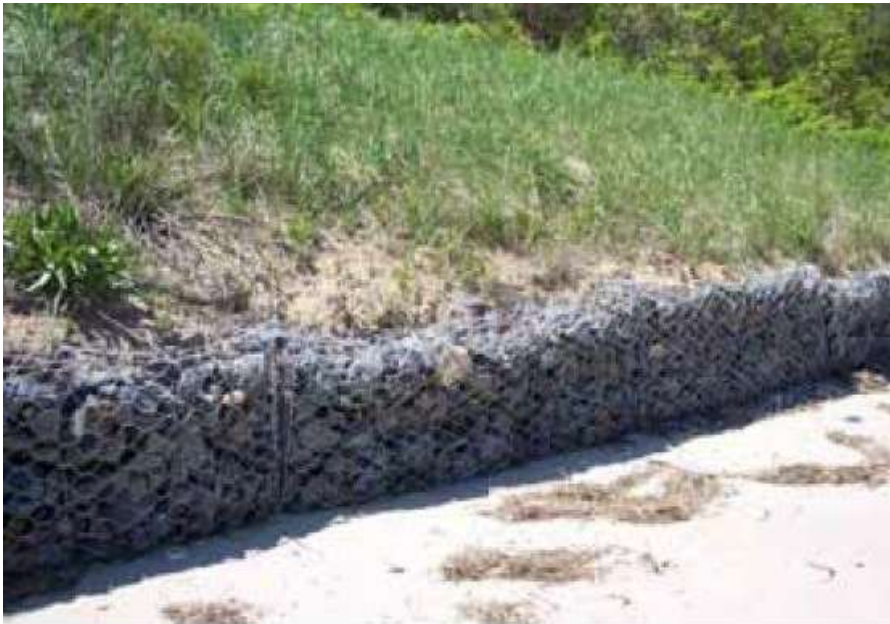
Image by K. Andres. Gabions installed in Chatham, MA.
