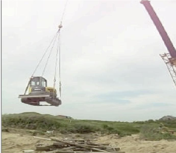
Prior to actual de-construction, confirm removal of household materials (liquids, furniture, appliances, carpets, paints and fuels) to minimize unexpected clean up. Wood bracing and small equipment can be delivered by crane.
