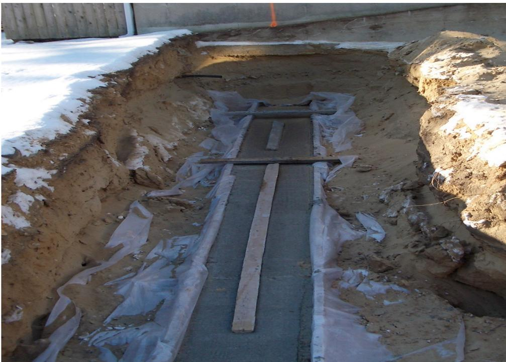
Liners create a stronger set by retaining moisture and act as a vapor barrier, which excludes ground moisture from the concrete structure.
