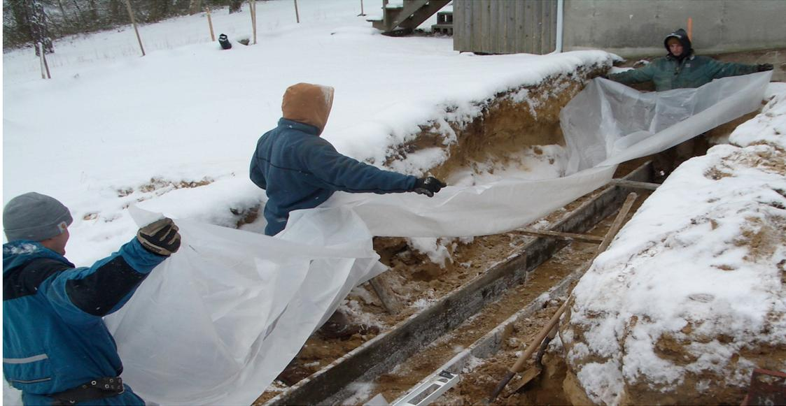
Inexpensive polyethylene liners under footings and slab forms protect ground water pH by preventing alkaline percolation while also providing a moisture barrier.
