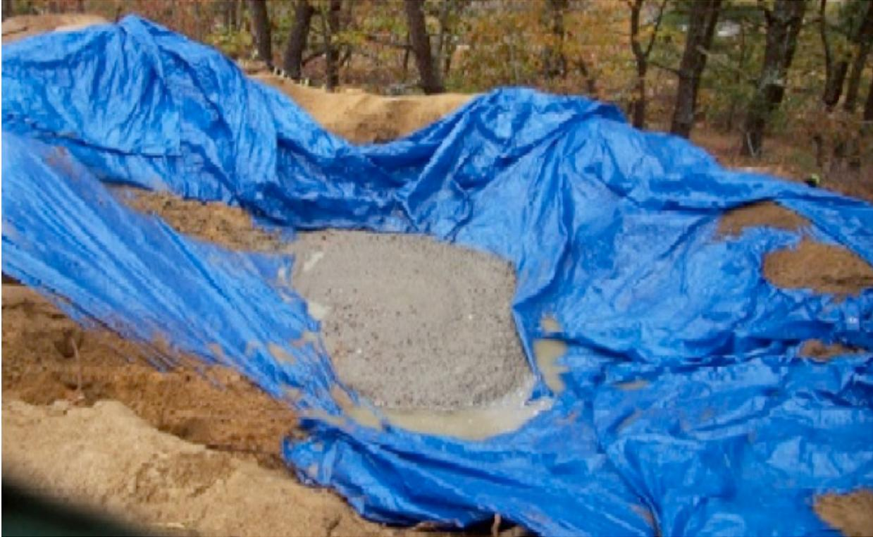
Pump trucks can utilize a large tarp dug into a backfill pile for excess concrete.
