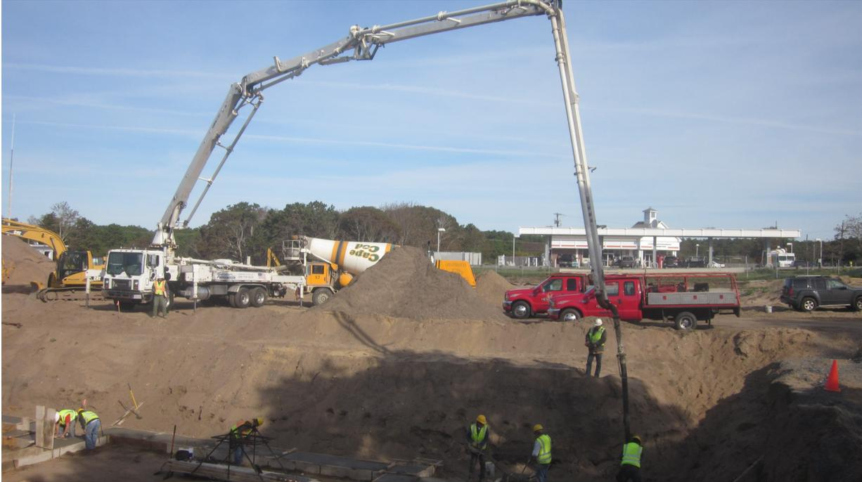
Site access may require distance delivery, with a concrete truck and pumper truck.
