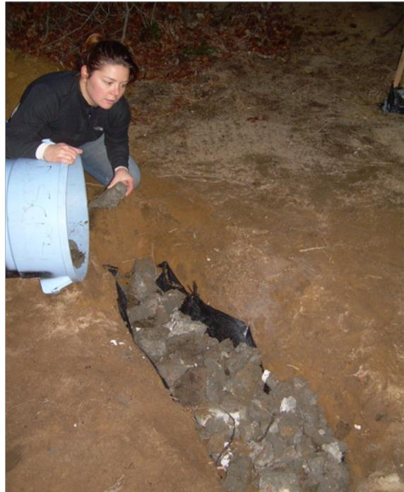
Over-pour should not be viewed as a waste product, but as a resource. After it has set, it can be broken up with a sledgehammer and used as fill for dry wells.
