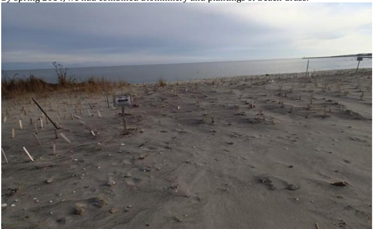
By late fall of 2014, there was enough sand captured by Biomimicry from storm over wash events to begin creating a barrier dune. Since this was a remote site, we used a boat for access. We adjusted the Biomimicry system when possible but were closed out by months-long sequences of winter storms, ice, and historic snow levels. We had no idea what we would discover, or what would remain, until we finally had a chance to return.
